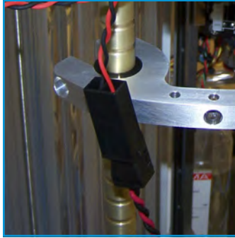
Figure 1-6: Power cable connected to ESP
